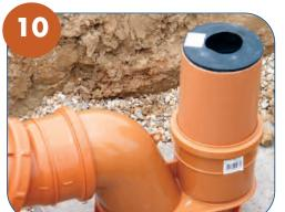
Rainwater downpipes connect to the system via a Universal Rainwater Adaptor.
