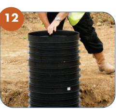
To complete the installation of Inspection Chambers, add risers to the required depth.
