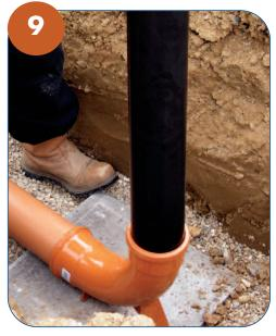
Soil and ventilation pipes connect straight into the long radius bend.
