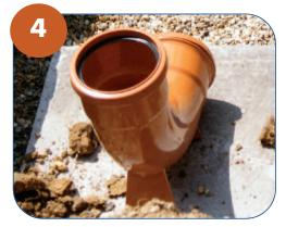
If fitting to a vertical soil and ventilation pipe, it is important to place a solid support under the long radius rest bend.
