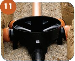
Install inspection chambers wherever there is a change of direction or a junction.
