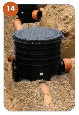
Backfill with pea shingle up to the crown of the pipework, and then backfill using the dug out soil.
